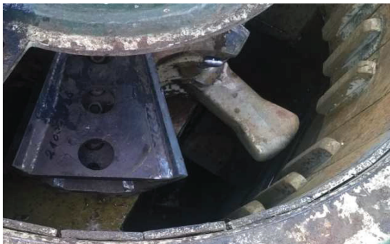
Fig 4. Distance between fix part and hammer, original (operational photo)
